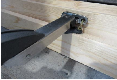
Flex window stay for top hung window
