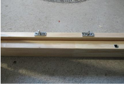
Screw extender to the casement
