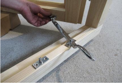
Screw extender to the casement
