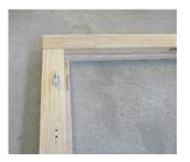
Install frame in wall and after that finish on inside with the 3 slats
